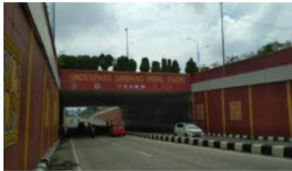
Gambar 1. Underpass Simpang Patal
