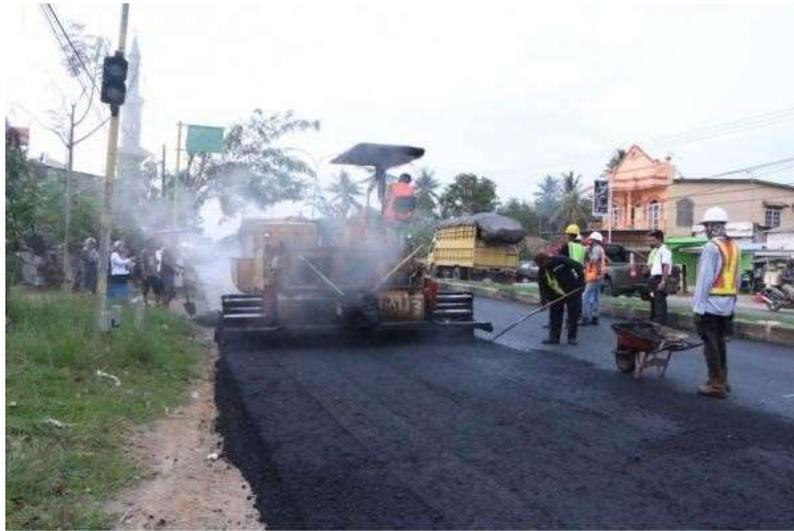
Gambar 2. *Cold Paving Hot Mix Asphalt (CPHMA)*
